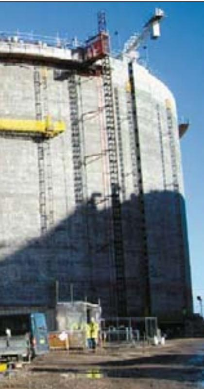
**1.** From January 2006 to February 2008, Freyssinet installed the prestressing of three new LNG tanks on the Isle of Grain (south east England).
