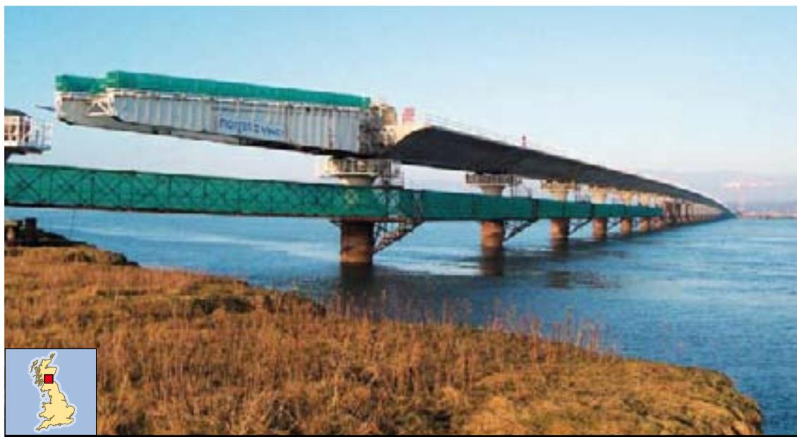
the “centered” temporary prestressing had to be installed: 94 m long rectilinear cables making up both spans. After the launching, the teams then installed the continuity prestressing using 140 m cables. The carefully prepared installation of the
