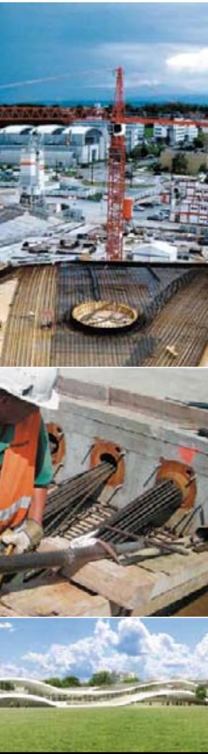
work, forming special concrete and developing a “hybrid static system”, where some shells act as tied arches, while others bear on these arches while retaining their function as a shell.
