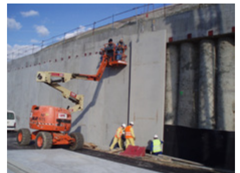
M-50 Highway (Madrid – SPAIN) - Abutment pile coverings
