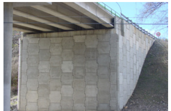
Reinforced earth abutment, supporting I beams
