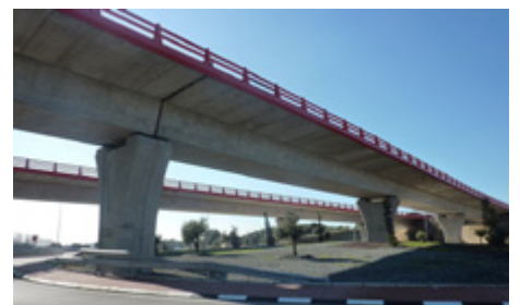
M-503 highway - Viaduct over Guadarrama river (Madrid - SPAIN) - Curved alignment solved with straight wide 1.50 m high U mono-beams
