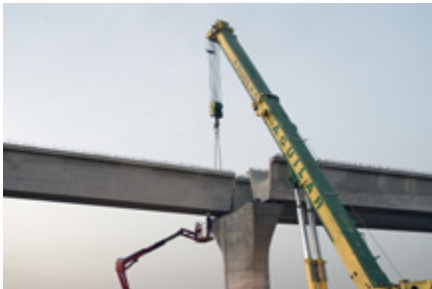
High Speed Train Viaduct - Section Mocejón - Toledo (SPAIN) Spans length: 36 m - 2 narrow TA-260 beams per span
