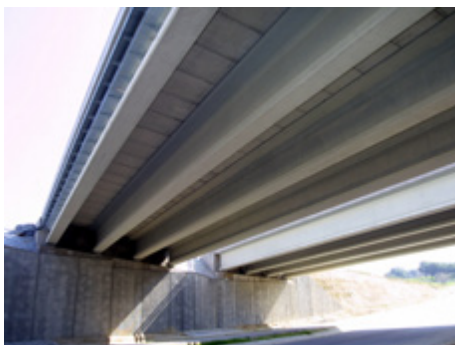
M-501 Road duplication (Madrid – SPAIN) - Buttressed panel abutment
