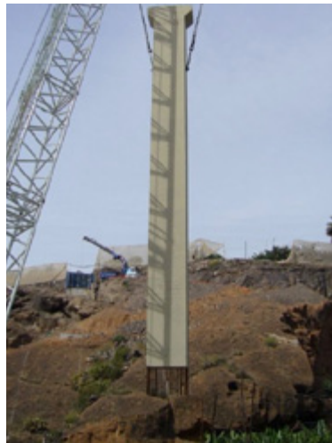
Water and gas pipeline bridge in Adeje (Tenerife, Canary Islands - SPAIN) - Hollow piers; transversal section 1.50x2.20; height 30.0 m
