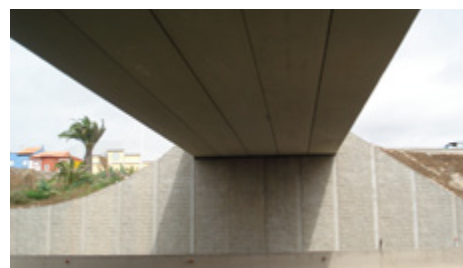
Bridge over the TF-1 Highway, Tenerife (Canary Islands - SPAIN) - 4 TPP 165.180 beams per span
