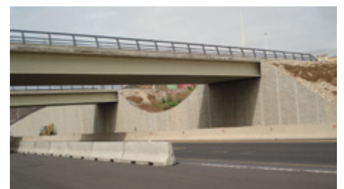
Bridge over the TF-1 Highway, Tenerife (Canary Islands - SPAIN) - 4 TPP 165.180 beams per span
