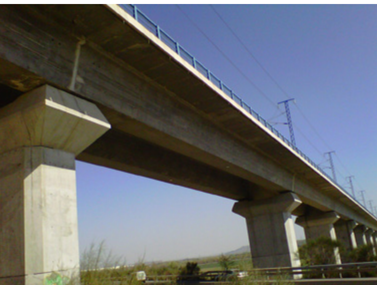
High speed train line Madrid – Barcelona (SPAIN) - Spans length: 30 m - Beam height: 1.90 m - Beam-to-beam joint detail
