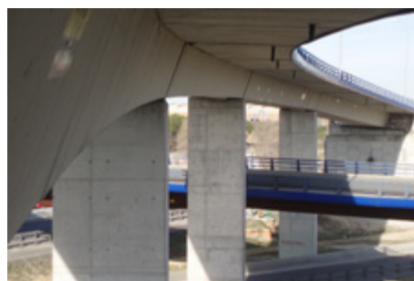
Curved highway connection, from M-45 to A-2 (Madrid - SPAIN), solved with a curved wide 1.50 m high U mono-beam
