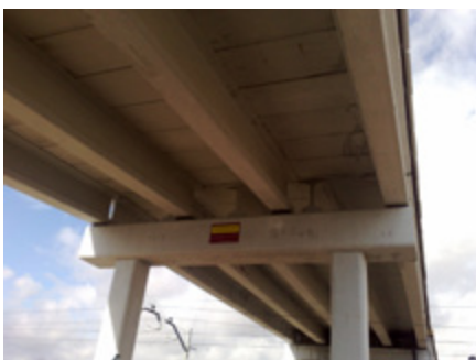
Bridge over Madrid-Guadalajara Railway (SPAIN) 4 IL-110 beams per span
