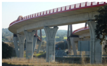
M-503 highway - Viaduct over Guadarrama river (Madrid - SPAIN) - Curved alignment solved with straight wide 1.50 m high U mono-beams
