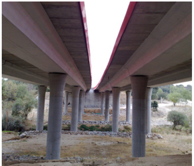
M-503 Highway - Viaduct over Aulencia river (Madrid - SPAIN) - 2 narrow TA-110 beams per span, supported by circular piers
