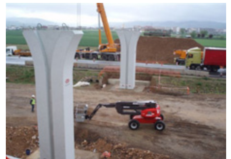
A-12 Highway (Camino de Santiago Highway) Hervias-Grañon section (La Rioja - SPAIN) Deck supported by palm shaped precast piers
