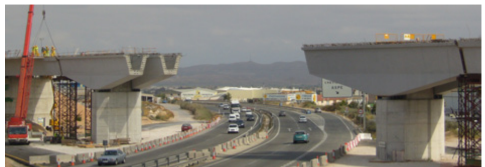
Baladrés Viaduct - Hyperstatic section over A-31 Highway (Alicante) - Spans length: 40 - 62 - 40 - Beam height: 2.60 m - 4.60 m
