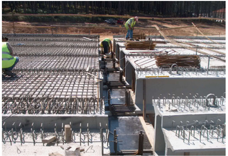
IP-3. Scut Interior North (PORTUGAL) - Construction of an in situ transversal beam, in an hyper-static I beam deck
