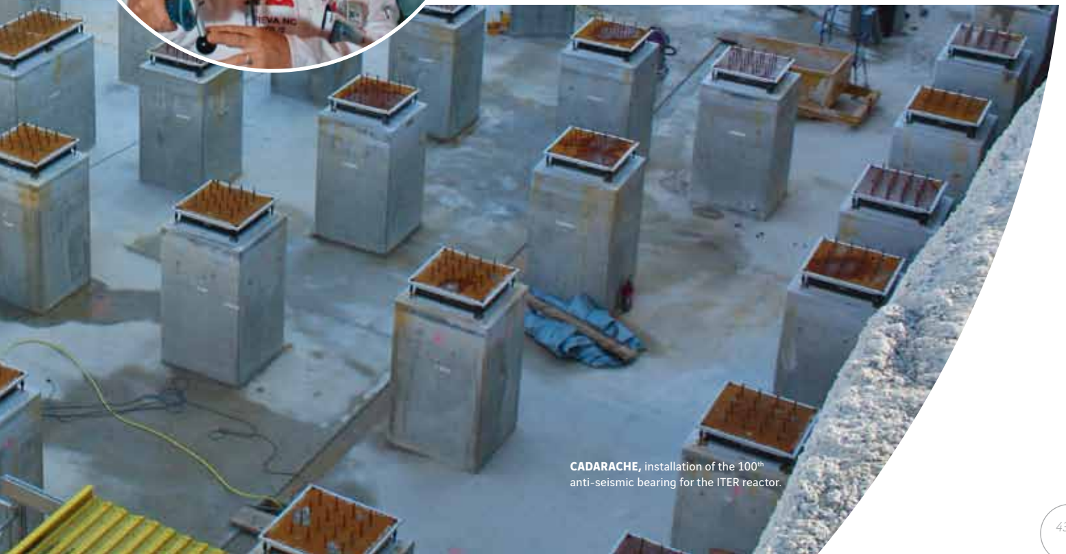
Remote operation Areva La Hague, Salvarem team, France.
