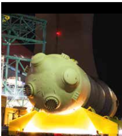
Steam Generator Replacement – Cruas-Meyssse
