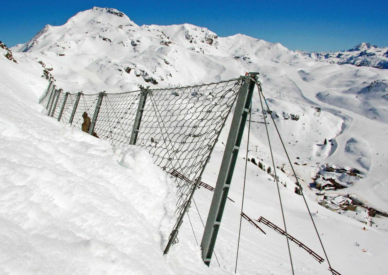
Snow nets prevent the development of avalanches by giving structural support to the snow mass in initiation zones having medium to large snow depths. This is in contrast to other approaches such as artificial release methods - e.g. using explosives - that initiate smaller avalanches before the hazard grows to an unmanageable size.
