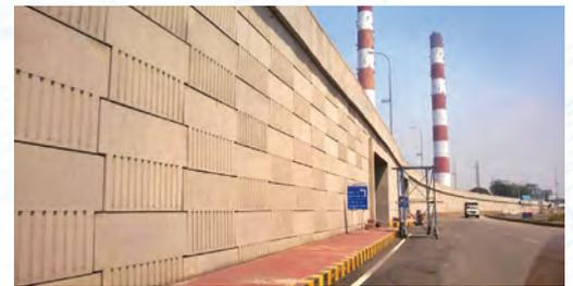
**Reinforced Earth®** structures combine engineered backfill with steel or synthetic tensile reinforcement and a modular concrete facing system. This ideal combination creates a durable and resilient earth retention structure. With **Reinforced Earth®** structures we can create several attractive architectural finishes.
