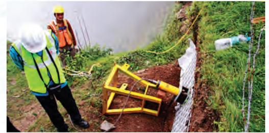
**TerraAnchor™** technology is an active soil reinforcement system used for permanent as well as temporary stabilization of existing slopes / structures by using high tensile steel as soil reinforcement (galvanized bars for permanent and strands for temporary). It is a driven and stressed soil anchoring system used with suitable facing.
