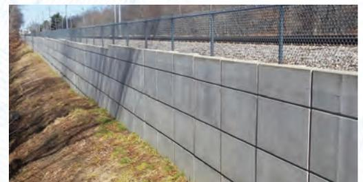
The **T-Wall®** system is a precast modular gravity type reinforced concrete retaining wall system. It is most suited for railway load supporting structures and construction of submerged retaining structures. The **T-Wall®** system decreases in stem length course by course – reducing materials, excavation and backfill as compared to other wall systems.
