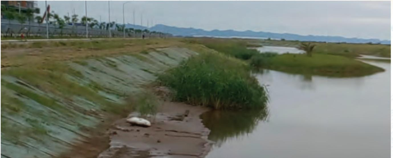
**TerraGreen®** is a custom designed erosion control mat / blanket useful for protecting dry and intermittently wet and erodible slopes. **TerraGreen®** as a stand-alone technique or mixed with other solutions like TerraNail® or TerraAnchor™ and high-tensile steel netting is often used to mitigate low to medium grade surface erosions and soil slips and slides.
