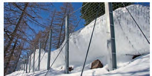
**Avalanche Barrier** systems are designed on a site-to-site basis to protect infrastructure, utilities, buildings, reforestation, and lives from avalanches. Snow nets, snow rakes and steel snow bridges are installed in the initiation zones to prevent avalanches from forming. Static defense structures, snow catchment fences/ barriers are used which effectively reduces the run-out length of an avalanche.
