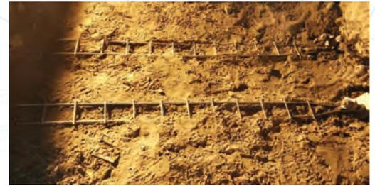
**ReMain®** is a specific selection of techniques used to maintain, strengthen and upgrade Reinforced Earth® structures. **ReMain®** is used for restoration and strengthening of existing structures (typically retaining structures, bridge abutments, wing walls and return walls). The durability, service life and performance of the affected structure can be significantly improved.
