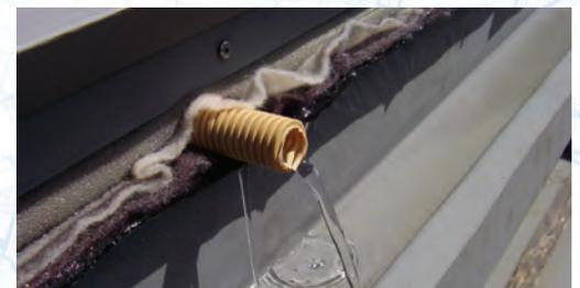
**DRAINTUBE™** has unique benefits over other geocomposite drainage systems; such as no geotextile intrusion, no creep and no peel adhesion issue. These ensure long term performance in most difficult conditions. Each roll performs the functions of separation, filtration and drainage.
