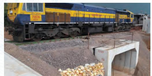
**TechBox®** is a state-of-the-art precast 'box' structure, typically a one- or three-segment system suitable for cut 'n' cover buried structures. The precast segments are brought to the installation site, when the site is ready for construction. It allows rapid on-site regulated installation. The soil cover required in **TechBox®** structures is lower than for arch structures.
