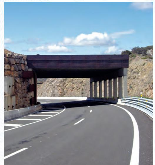
Rockfall is an inherent hazard of mountainous terrains, which jeopardizes life, property and threatens the smooth operations of traffic lines. **TechShelter®** is a perfect custom-designed solution of pre-cast arch box (TechBox® and TechSpan®) for sheds and shelters to suite these site conditions. This is one of the most reliable, cost-effective system for cut 'n' cover structure.
