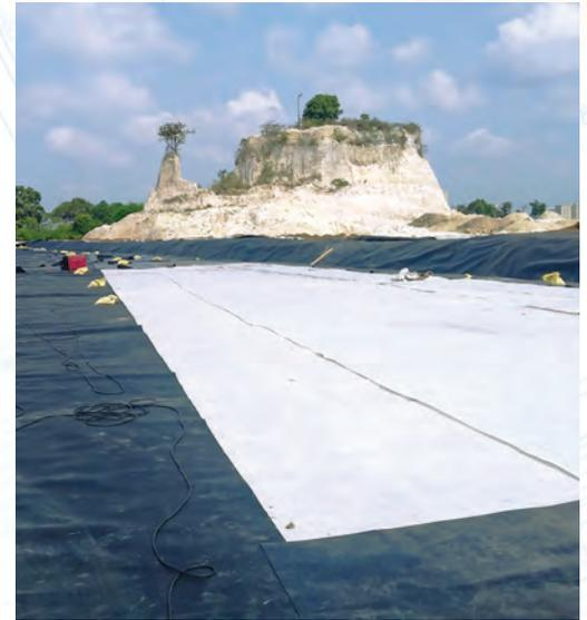
**TerraLine®** Geosynthetic Clay Liners (GCL) are factory made hydraulic barriers consisting of very low-permeability bentonite powder supported by geotextiles and/or geomembranes. The engineering function of a **TerraLine®** – GCL is containment as a hydraulic barrier to water, leachate or other liquids and sometimes gases.
