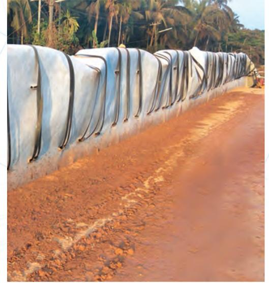
**TerraFlow®** Geocomposite consists of bi-planar High-Density Polyethylene (HDPE) geonet having non-woven polypropylene (PP) geotextile heat bonded on both sides. Bi-planar geonet is designed with two HDPE strands crossing each other at a constant angle to form a diamond structure to provide better planar waterflow under high loading. Tri-planar geonet consists of three HDPE strands to improve the lateral drainage and transmissivity.
