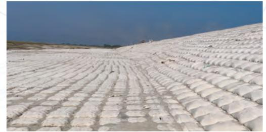
**TechRevetment®** is a pre-engineered factory costumed grouted mattress system used for permanent erosion protection works. This technology is used to protect embankments, protect bridge abutments against scour, for bed protection of major rivers and waterways, and for shoreline protection. This system can be installed at rapid speed and under water without the need for dewatering.
