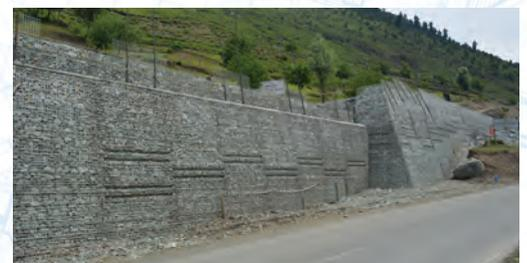
Hilly terrains infrastructure are often prone to landslides, steep slopes, rockfall and debris flow. Terre Armée India offers bespoke **Reinforced Earth® Steep Slope** technique to build steepend slopes for slope engineering and geo-hazard solutions. **Reinforced Earth® Steep Slope** technique uses both mineral and vegetative facing finishes that appropriately blend with project requirements.
