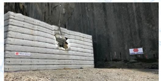
**TerraBund®** is a Terre Armée protection bund. It is a gravity structure built using soil reinforcement and flexible or semi-rigid facing systems. It is a passive protection system used typically as a geo-hazard solution against rockfalls, avalanches, debris flow and mud slides. **TerraBund®** can withstand more than 8000kj of impact energy in the event of landslide or rockfall.
