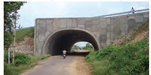
**TechSpan®** is one of the most reliable, cost-effective precast concrete arch systems available for cut 'n' cover structures. It is widely used in the construction of bridges, underpasses, conveyance and reclaim tunnels, portals, ammunition storage bunkers and rockfall sheds and shelters. Typically, 15-20 linear meters of **TechSpan®** can be installed in one work shift.
