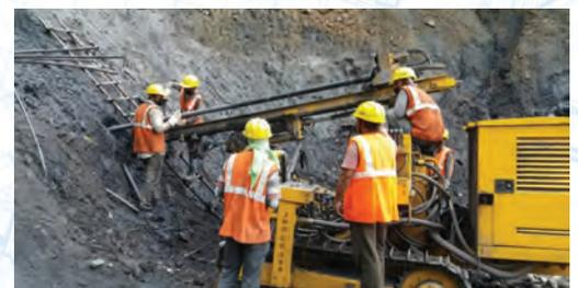
**TerraNail®** is an in-situ method of reinforcing existing soil/rock mass by installing solid or hollow fully threaded hot-dip galvanized high tensile geotechnical steel bars encased in grout. **TerraNail®** is typically used to stabilize existing slopes or excavations. It is also a reliable solution for landslide rehabilitation and active rockfall protection.
