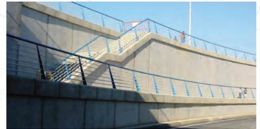
**TechWall®** precast retaining walls and abutments are effective solutions when a standard footing is used or when site conditions rule out the use of Reinforced Earth® structures. **TechWall®** is developed as an engineered product with low lifecycle costs and long-term performance, which helps minimize overall construction duration and reduces site works.
