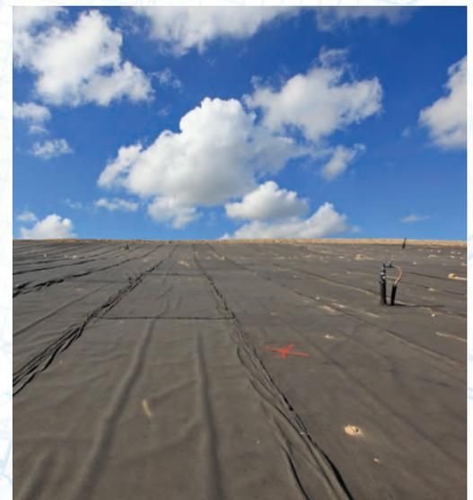
**TerraTextile®** is a specially made technical textile, either woven or non-woven. They offer excellent strength and hydraulic characteristics; and cater for a wide range of applications. **Woven TerraTextile®** is used for soil reinforcement, separation and filtration, secondary reinforcement, erosion control, ground stabilisation, silt fence etc. **Non-woven TerraTextile®** is very popular in applications such as filtration, separation, sub-surface drainage and transmission erosion control.
