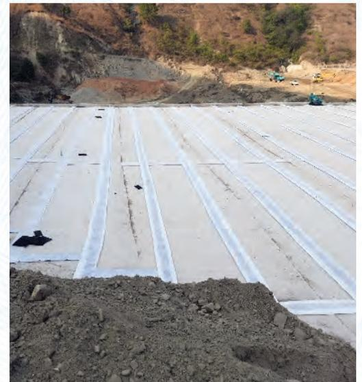
**TerraDrain®** is modular light weight, high strength and high impact cellular drain board wrapped with a custom designed geotextile and used for subsurface drainage. The drainage board and the non-woven geotextile used in **TerraDrain®** are manufactured from polypropylene. The open surface design and high internal void volume enables the rapid capture and transport of high amount of water.
