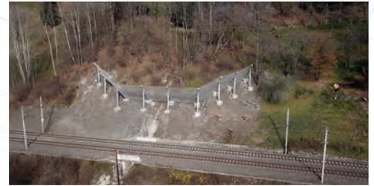
Terre Armée offers engineered solutions to protect infrastructure, and assets from debris flows and debris floods. The threat of climate change raising the global temperatures, potentially causes a change in weather patterns, thawing of permafrost areas, increasing wildfires, debris flows, and shallow landslide activity. The use of flexible-net barriers can be an efficient alternative to the other traditional and costly mitigation measures such as dams and other rigid barriers.
