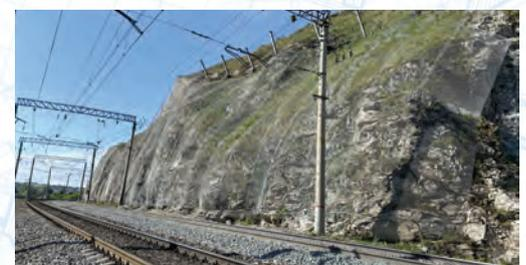
Terre Armée offers engineered solutions for **Slope Retention** to retain the masses in situ and prevent erosion and shallow landslides. This systems is designed on a site to-site basis. Depending on the site characteristics and strength requirements, a large variety of net and netting products are available. Re-stabilization of the slope using mesh and natural vegetation is highly encouraged. Furthermore, netting can accommodate pre-existing vegetation such as tree trunks with minimal effort.
