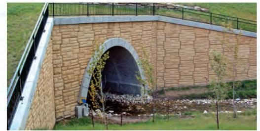
**TechCulvert®** is small to medium sized single unit Precast 'Box' or two-pin Precast 'Arch' for hydraulic culverts and utility covers (like gas pipelines). **TechCulvert®** provides several benefits to project owners, like assured quality, savings in indirect cost, rapid construction and early traffic commissioning.
