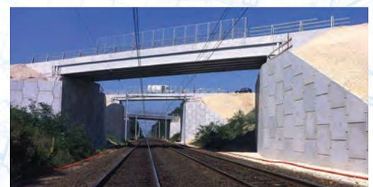
**TechAbutment®** is an alternative solution for RCC / piled abutments. A highly engineered technique, it has been adopted throughout the world successfully for over 40 years. It is a Reinforced Earth® structure designed to support bridge load as an alternative to conventional RCC abutments. This is used for bridges, underpasses, flyovers, ROB's and RUB's.
