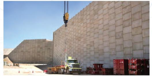
**Composite Earth®** technology adopts primary and secondary soil reinforcement systems for the design of Reinforced Earth® retaining walls. It aims to control the lateral deformation of the facing during construction and operation, including during seismic events. This is an effective way to design and construct tall and critical structures.
