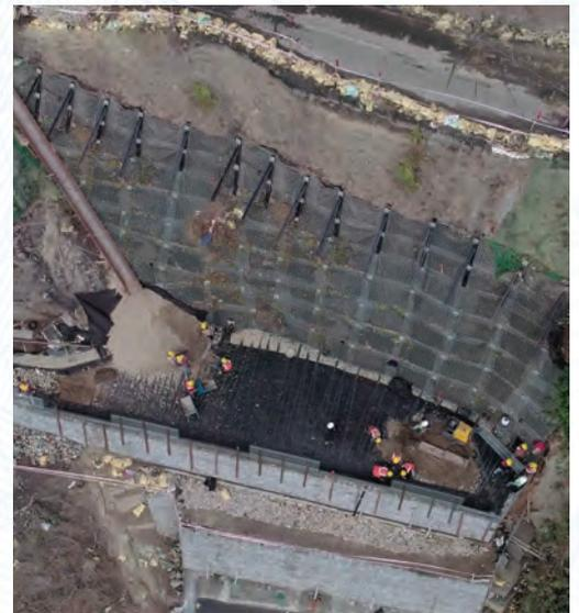
**TerraLink®** technique allows building of earth retention structures connecting existing profiles stabilized by soil nails and/or anchors. It is a useful technique for construction of benches and for road widening projects with limited available space, and activates the best optimisation between cut and fill requirements.
