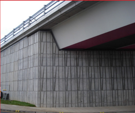
Access ramp to the London 2012 Olympic games site, United Kingdom
