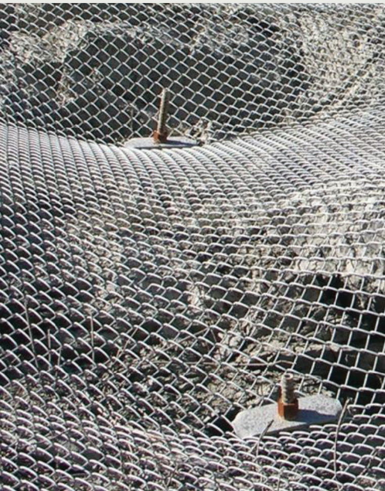
An example of interior anchors using a standard spike plate for the coupling. Anchor points are typically set in topographical lows whenever possible.
