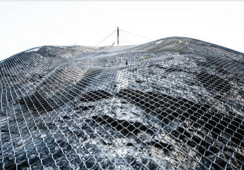
Rectangular netting lays flat against the slope and can conform to changes in topography better than hexagonal mesh.
