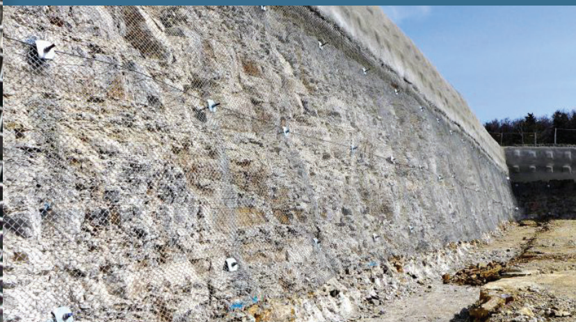
Rock wall reinforced using High Performance Netting.
