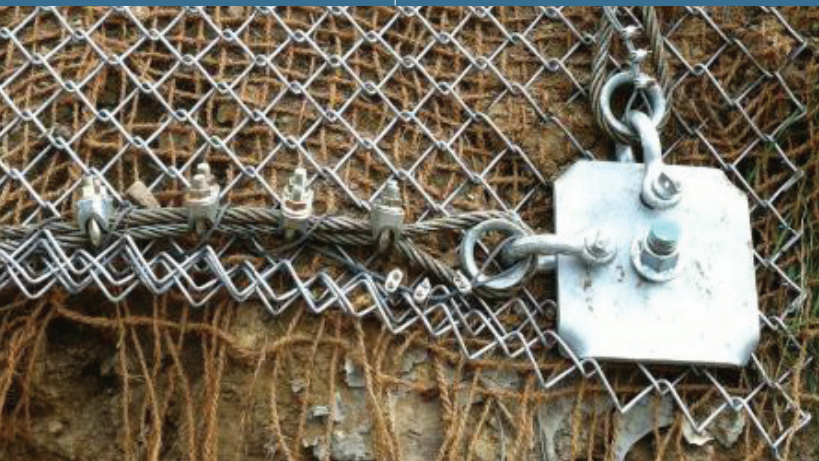
Corner plates are designed to receive bearing ropes using a shackle and thimble connection to ensure full strength and for ease of installation and maintenance.
